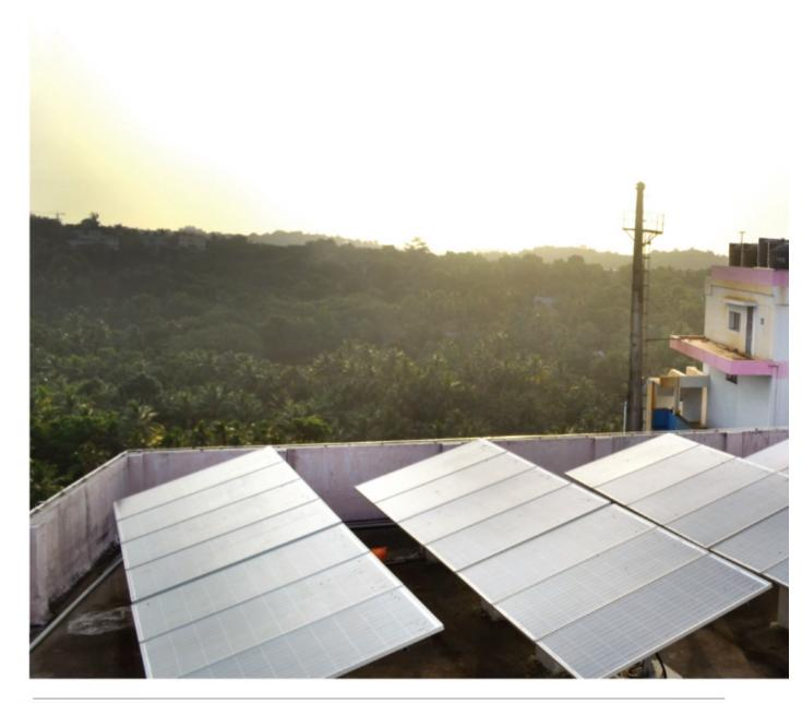
At a time when renewable sources of energy are much discussed as a solution to power crisis, HLL decided to take the lead and installed a 25 Kwp solar power unit at HLL's Akkulam Factory in Thiruvananthapuram (AFT).
